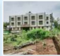
TRIBAL SCHOOL SUPPORT
